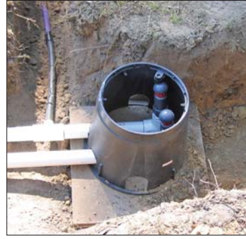
Installation of the dual-manifold air-vacuum relief valve and support block.
