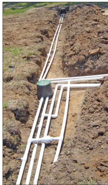
Above, the control panel rack, nearly finished. Temporary cords hanging from the panels were used to perform the inspection power-up. At left, trench installation for the subsurface drip distribution system and flush return manifolds for two of three zones.
