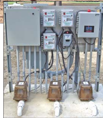
Above, the control panel rack, nearly finished. Temporary cords hanging from the panels were used to perform the inspection power-up. At left, trench installation for the subsurface drip distribution system and flush return manifolds for two of three zones.
