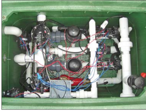
The JNM Technologies three-zone ACT C200S auto-flush filter system installation.
